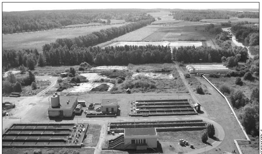
The 75-ha willow phytoremediation system at Enköping, central Sweden: wastewater treatment plant (foreground), ponds for winter storage of wastewater (background) and willow fields irrigated by wastewater from sludge
